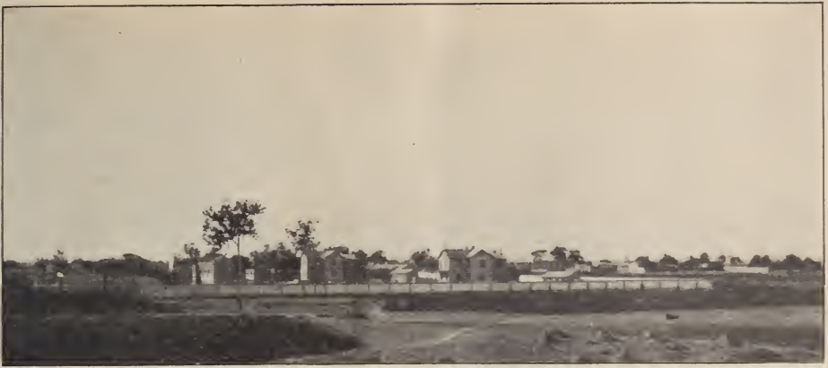
VIEW OF COMPOUND, LOOKING WEST FROM TOP OF CITY WALL
